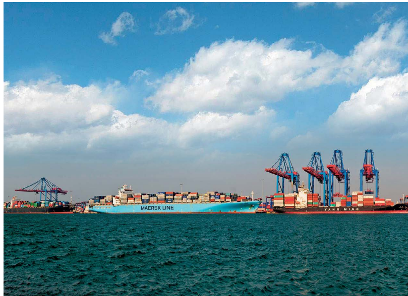
PORT SAID EAST CONTAINER TERMINAL - PHASE 2, MARINE WORKS, EGYPT
