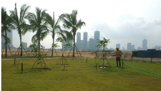
Landscaping for Phase I has commenced
